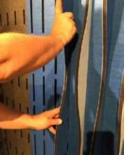
Attach BACK PANEL(S) plumb and touching to wall surface with (4-6) sheet rock screws (not included) through cut holes for each back panel or use construction adhesive if a masonary wall.
