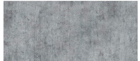
Y0374 Mack Ave Concrete
